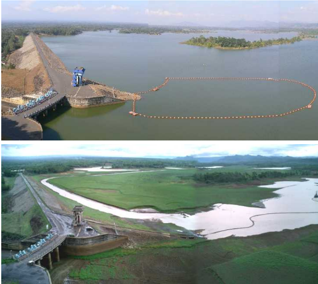
Figure 1 View of the Wonogiri Dam Reservoir during Normal High Water Level – 136 m (above) and Low Water Level - 127 m (below)
